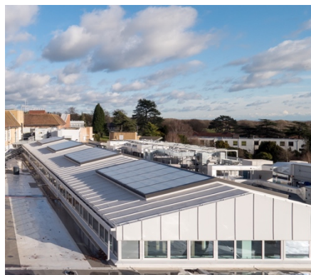
Typical translucent skyroof – exterior view
