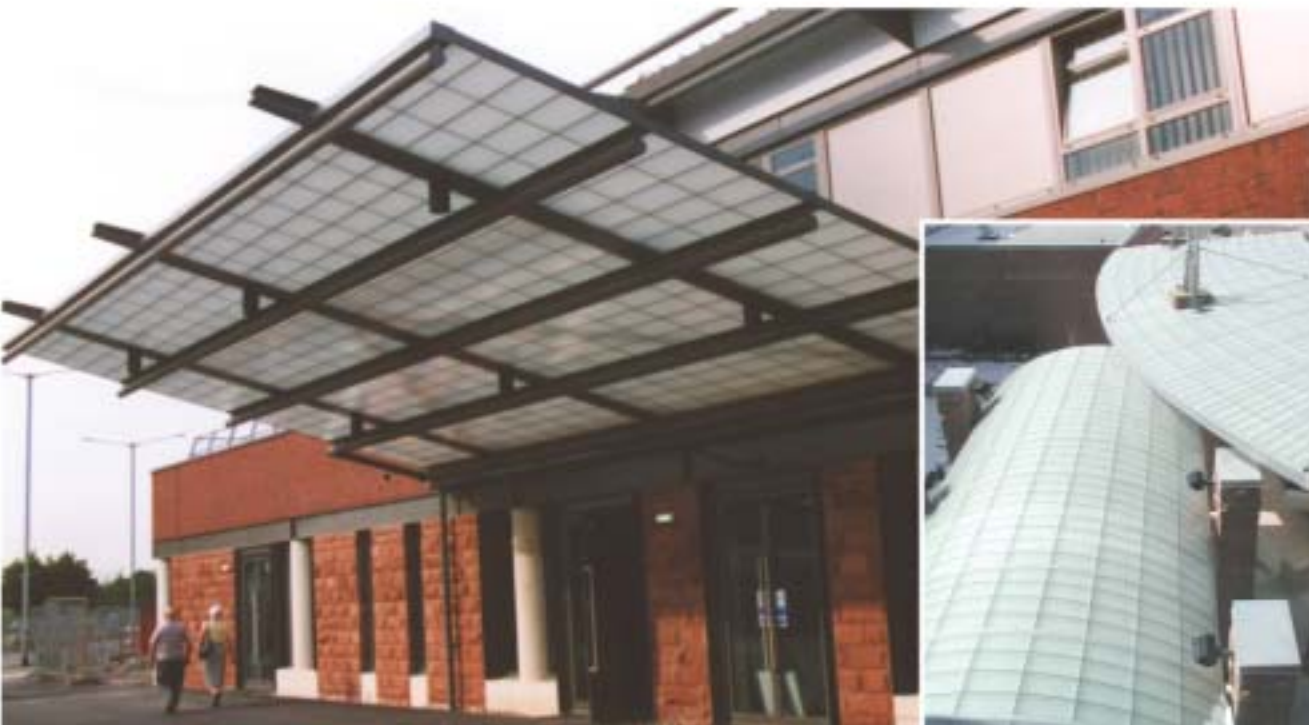
South Tees General Hospital, Middlesbrough, UK; HLM Architects
