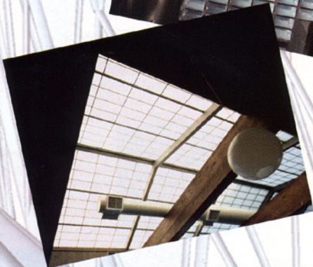
At 99.8 percent air, aerogel (top) is the lightest solid in the world; it will be used as a particle collector (middle) on NASA's Stardust mission; Cabot Corporation developed Nanogel, a translucent form of the material, which doubles the insulation in Kalwall day lighting panels (bottom).
